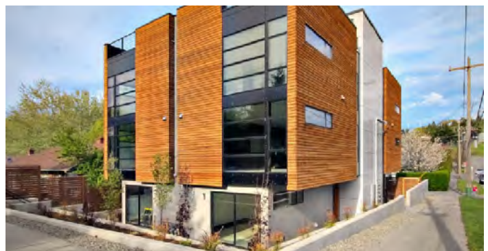
PB Elemental Architecture, Beacon Hill Washington
