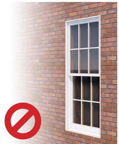
Flush Framing — Not Recommended
