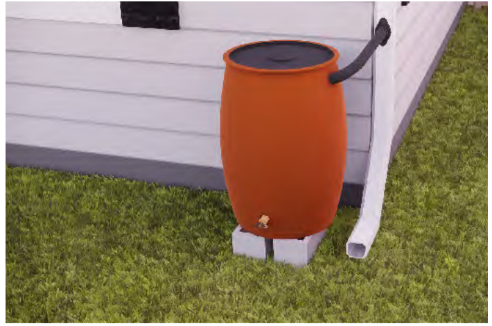
Rain barrel connected to a downspout
