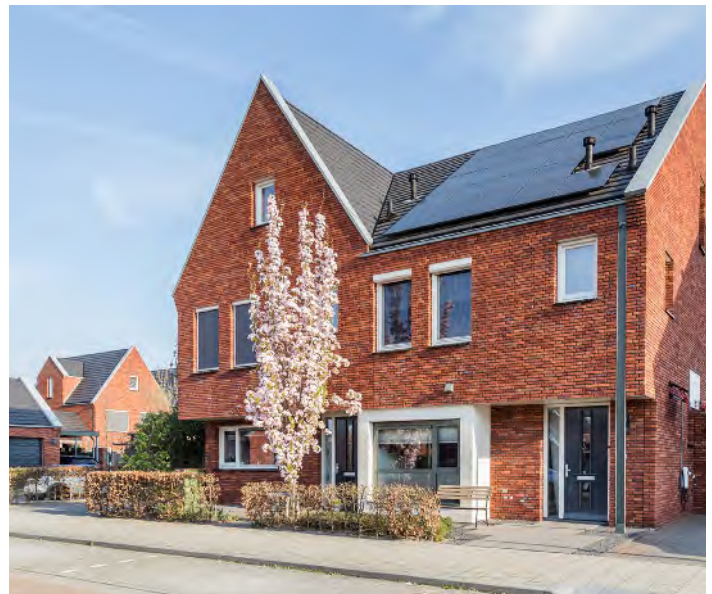
Solar panels installed on a duplex
