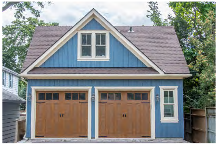
Chicago, IL — Heartland Garage Builders
