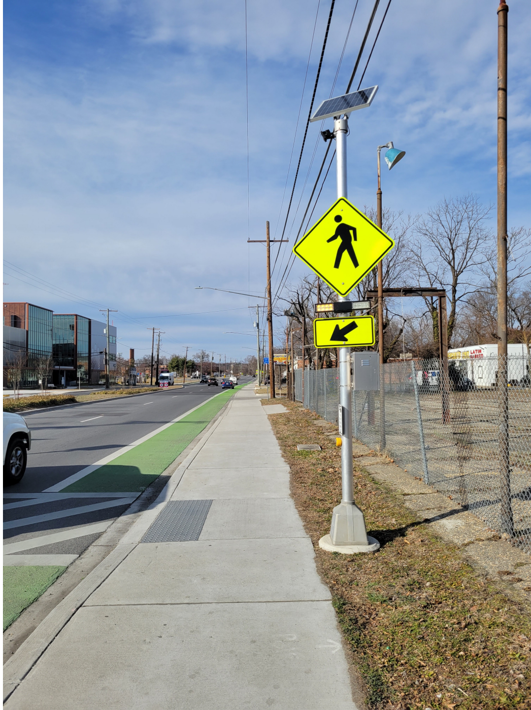
Facing North Rectangular Rapid Flashing Beacon (RRFB)
