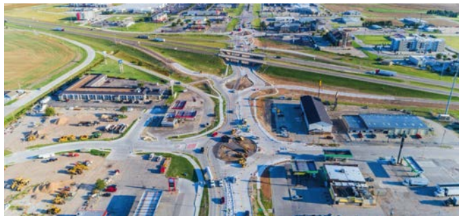
LOCATION: Vine Street (US 183), Hays, Kansas. SOURCE: City of Hays, Kansas.
