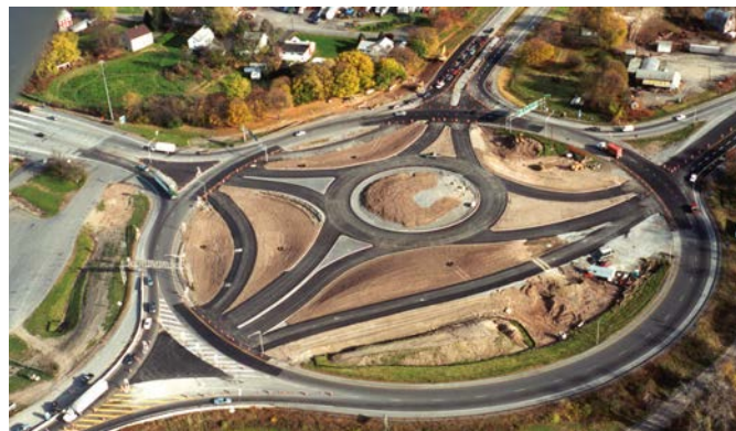
LOCATION: Albany Avenue/Broadway/I-587, Kingston, New York. SOURCE: New York State Department of Transportation, as shown in NCHRP Report 672 (1) .
