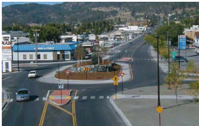
LOCATION: US 395 (Main Street)/E Hawthorne Avenue/Railroad Avenue/ S Washington Street, Colville, Washington. SOURCE: Brian Walsh.
