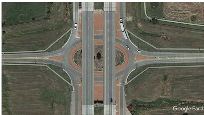
LOCATION: E Broadway Street/I-135 Ramps, Newton, Kansas. SOURCE: Google Earth.
