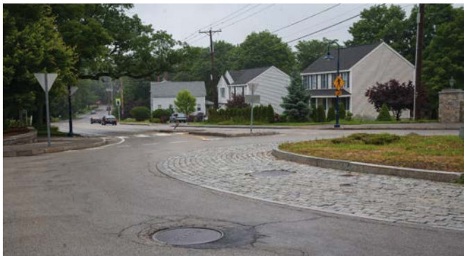
Exhibit 13.3. Example of flush truck apron using pavers.
