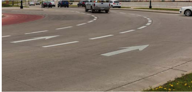
LOCATION: Mason Street / I-41 Southbound Ramps, Green Bay, Wisconsin. SOURCE: Lee Rodegerdts.
