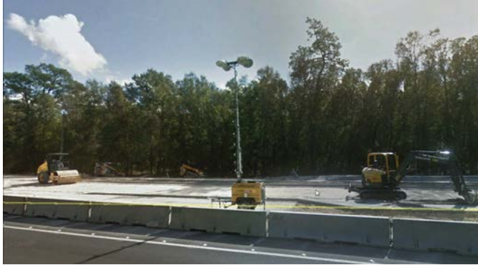
LOCATION: DeLand, Florida. SOURCE: Florida Department of Transportation.
