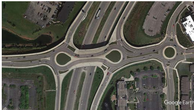
LOCATION: W Main Street/US 31 Ramps, Carmel, Indiana. SOURCE: Google Earth.
