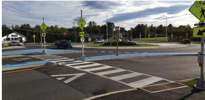
LOCATION: US 2 (Park Street)/Rangeley Road, Orono, Maine. SOURCE: Jonathan French.
