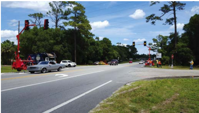
LOCATION: DeLand, Florida. SOURCE: Florida Department of Transportation.
