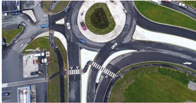
LOCATION: US 2 (Park Street)/Rangeley Road, Orono, Maine. SOURCE: Jonathan French.
