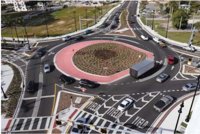
LOCATION: N Tamiami Trail/Fruitville Road, Sarasota, Florida. SOURCE: Ken Sides.
