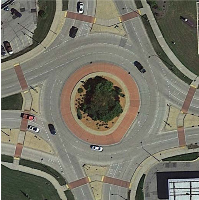
LOCATION: Shawano Street/South Taylor Street, Green Bay, Wisconsin. SOURCE: Google Earth.
