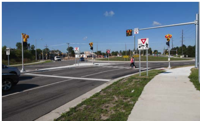
LOCATION: West Maple Road/Drake Road, Oakland County, Michigan. SOURCE: Lee Rodegerdts.
