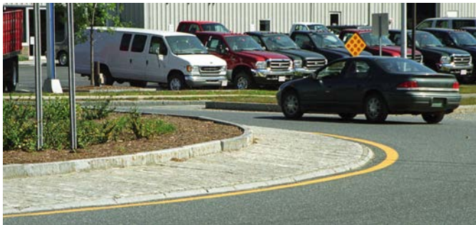
Exhibit 13.2. Example of raised truck apron using pavers.
