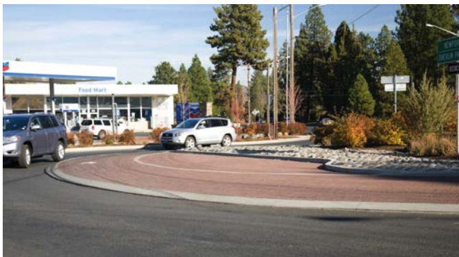
LOCATION: NW Shevlin Park Road/Newport Avenue/College Way, Bend, Oregon. SOURCE: Lee Rodegerdts.
