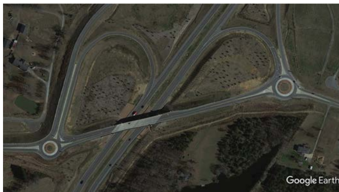
LOCATION: Austin Chaney Road/US 74 Bypass Ramps, Monroe, North Carolina. SOURCE: Google Earth.
