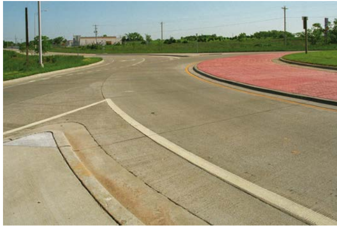
LOCATION: Rice Road/I-70 Eastbound Ramps/Cyprus Drive, Topeka, Kansas. SOURCE: Lee Rodegerdts.
