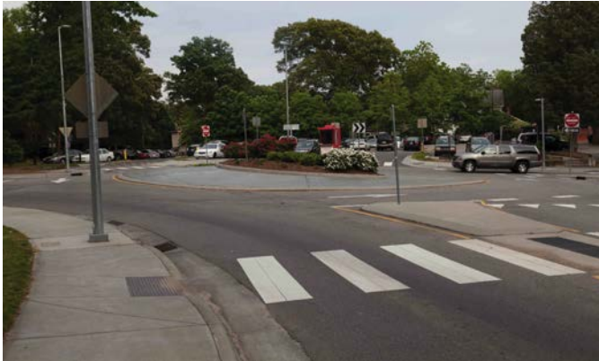
LOCATION: Oberlin Road/Pullen Road/Groveland Avenue, Raleigh, North Carolina. SOURCE: Lee Rodegerdts.
