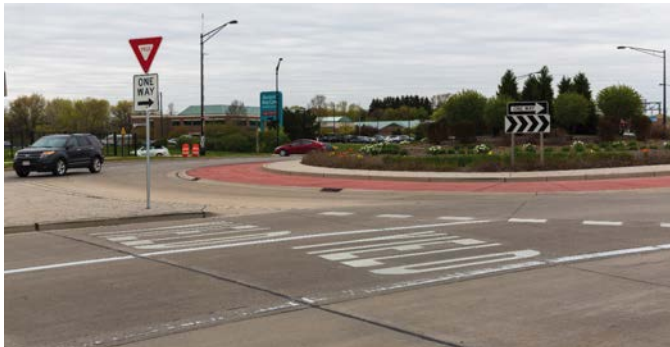
LOCATION: W Mason Street/I-41 Southbound Ramps, Green Bay, Wisconsin. SOURCE: Lee Rodegerdts.
