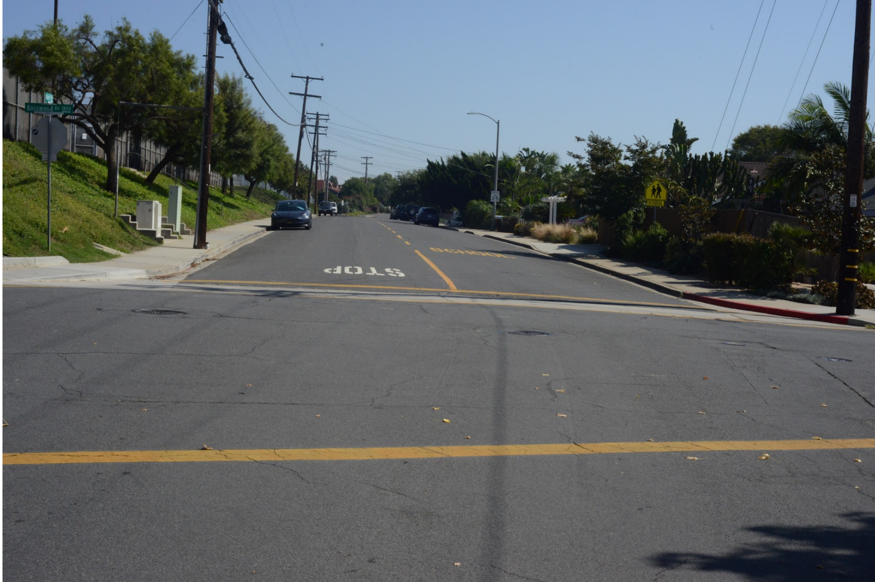
NW of Intersection Looking S/SE onto Valley
