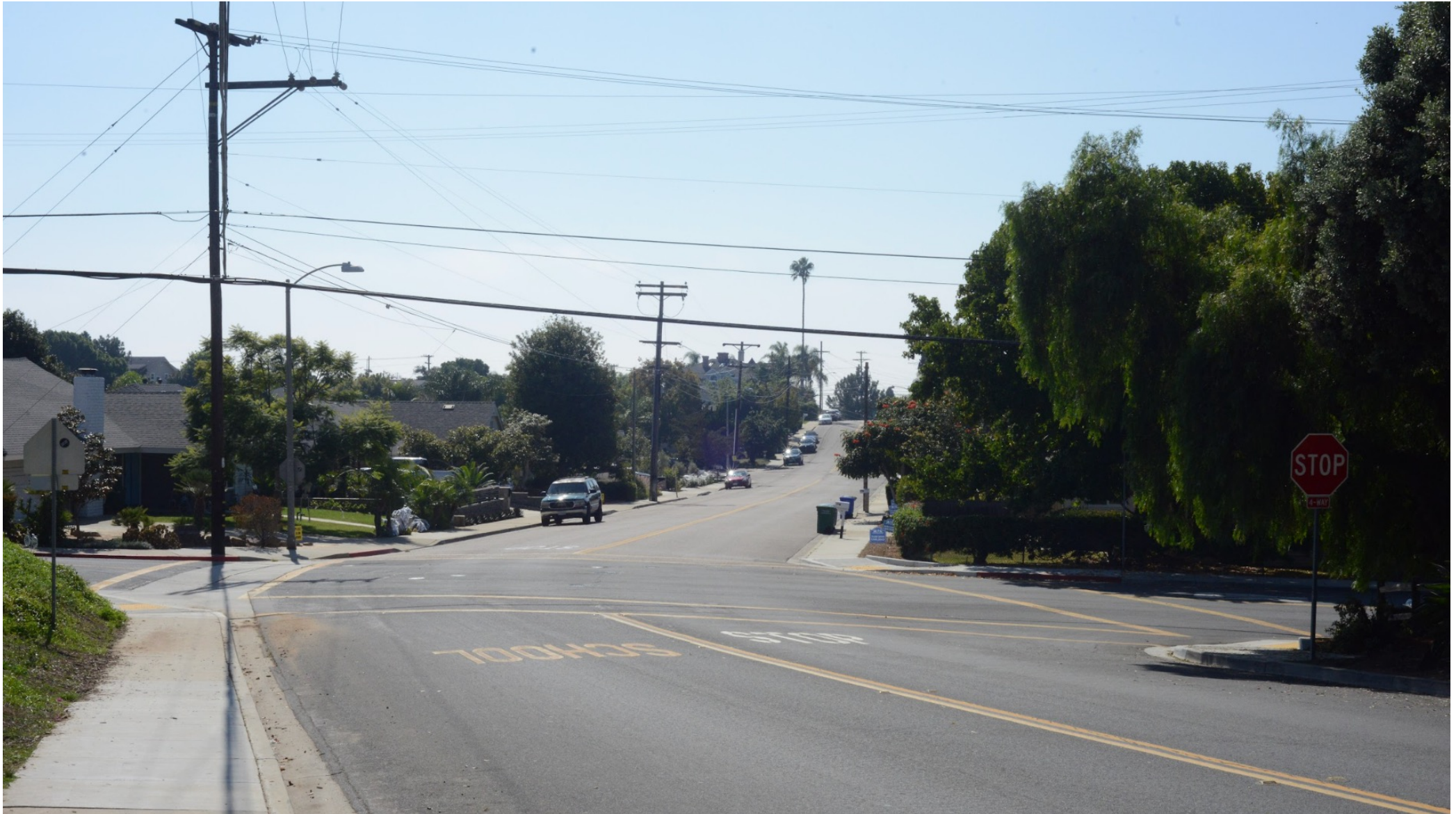
NE of Intersection Looking onto Basswood
