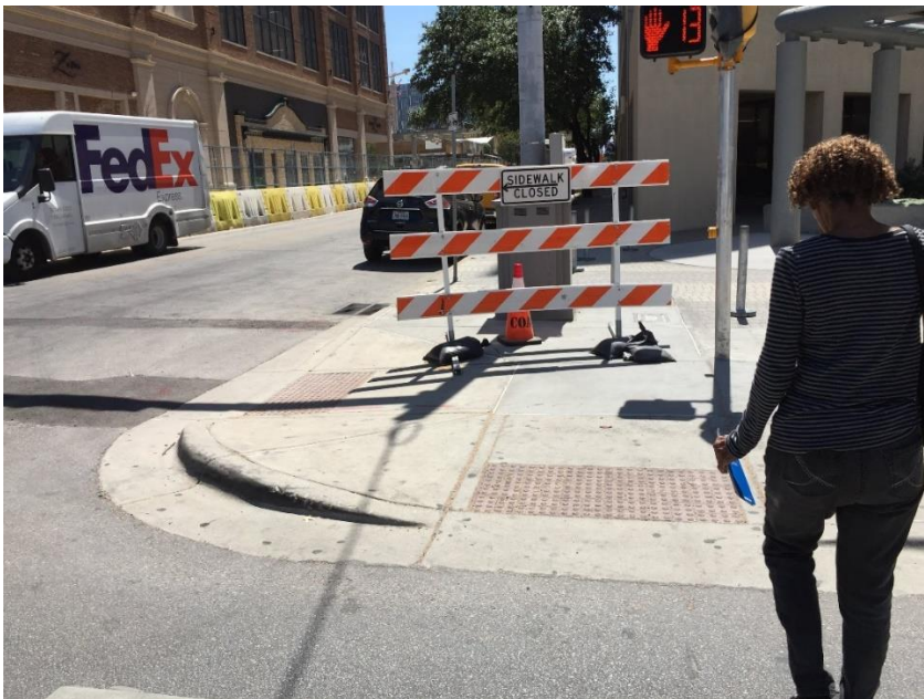
Photo of a sidewalk closed for construction by Heyden Black Walker
