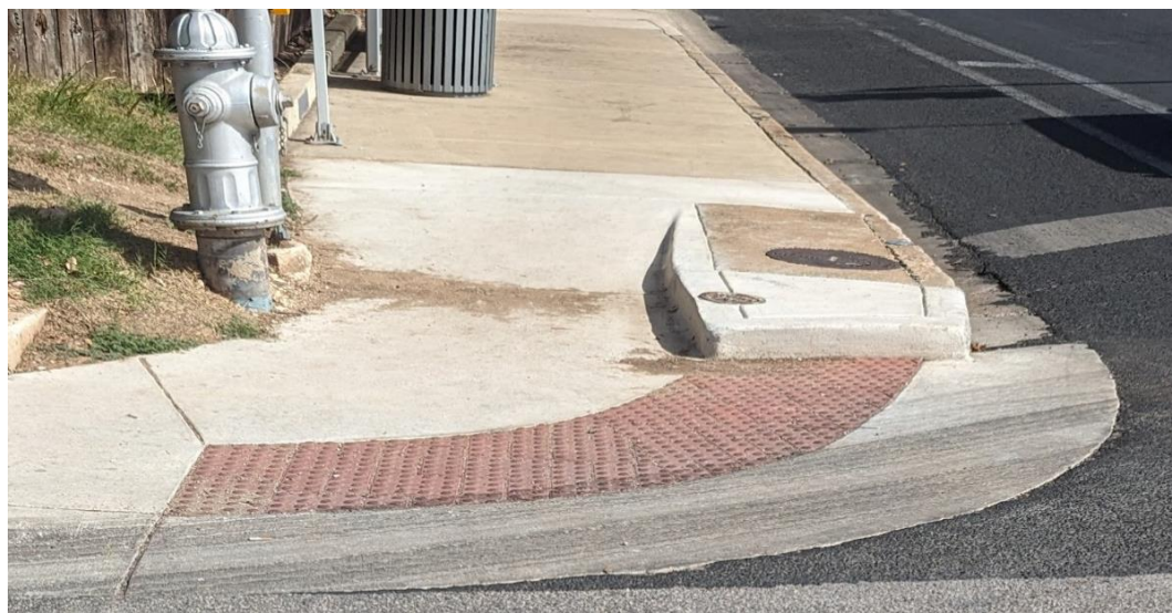
Photo of truncated domes on a curb ramp by Marissa Bell
