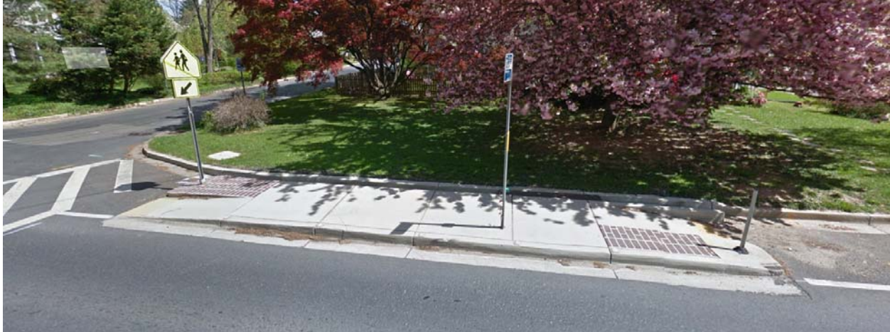
A bus stop in Silver Spring, MD. A sidewalk has been added in the shoulder only at the bus stop.
