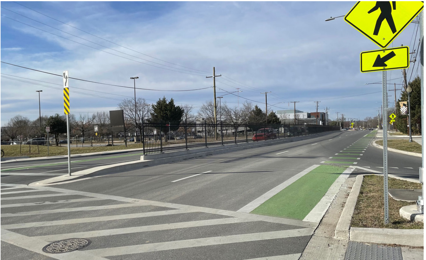
Ager Road approaching an intersection with Hamilton Street in Hyattsville, Maryland. Ager Road features wide automobile travel lanes, a slip lane to facilitate faster speeds for drivers entering the street, wide margins on either side of the road, and other design elements that induce travel speeds too fast for the urban environment.
