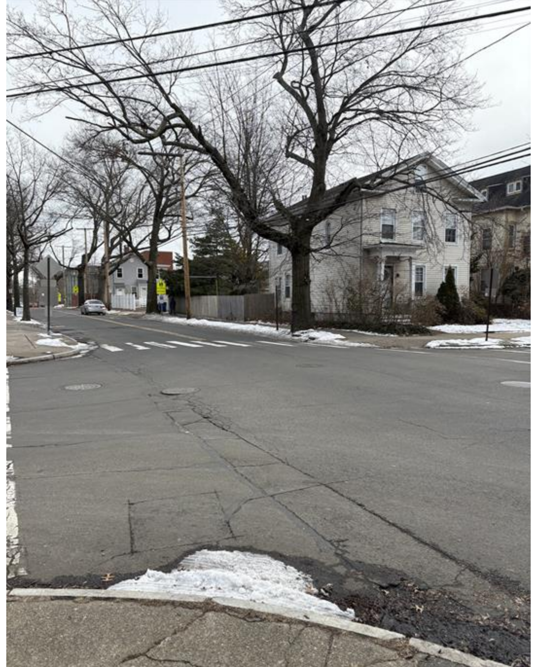
Intersection from NW Corner (looking SE)
